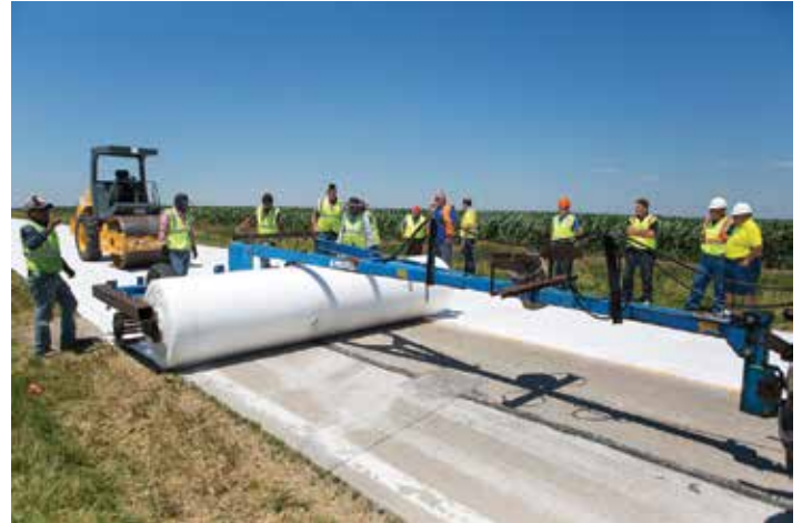
Jason Aschoff, Project Manager for A & R Construction held his crew around to show how easy the fabric is to place. Jason and his crew modified a farm implement to carry and unroll the fabric. Hand sprayers were used to apply the glue.
